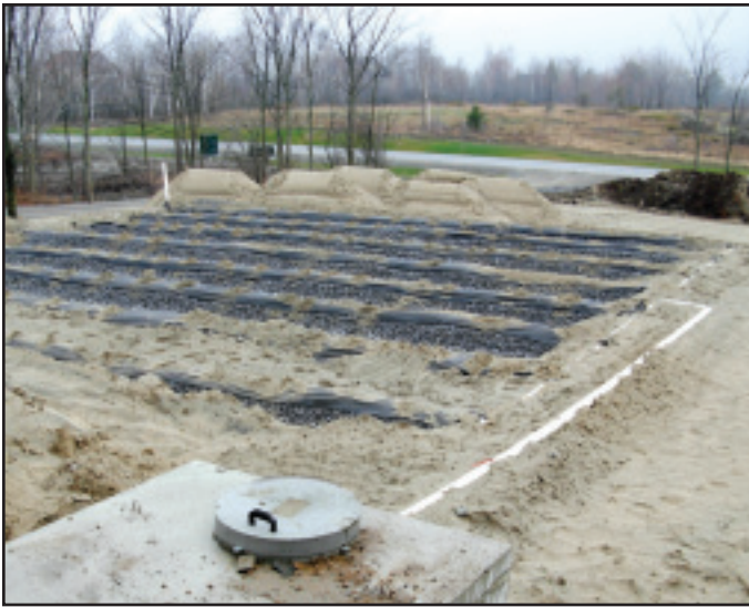
Leaching bed with perforated PVC drain pipes.
