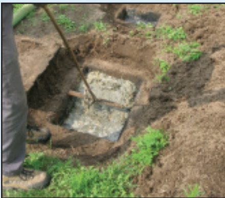
Scum level is too high. Time to pump your tank and inspect your leaching bed.
